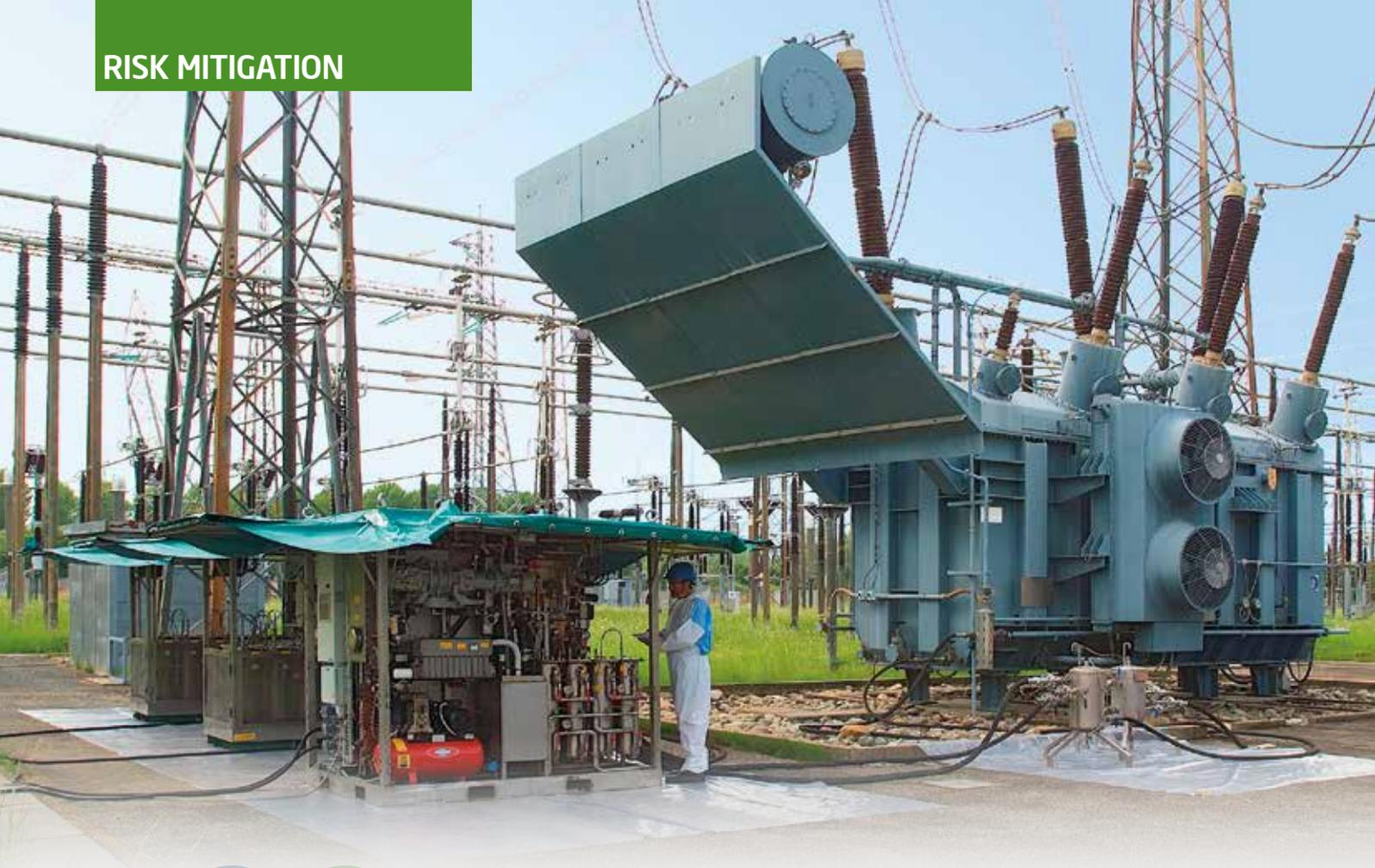
**Specific oil treatment may be performed keeping the transformer in operation, energised and loaded even in nuclear power plants and on transformers up to 780 MVA and up to 500 kV**
