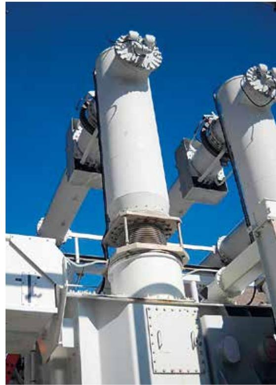
Figure 3. View of a CTzk bushing model
