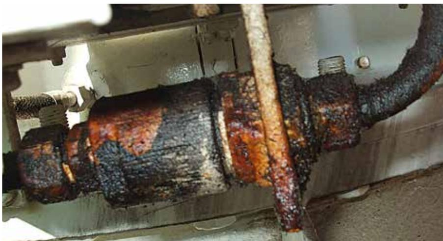
Figure 4. Rusty and leaking valve on CTG bushing
