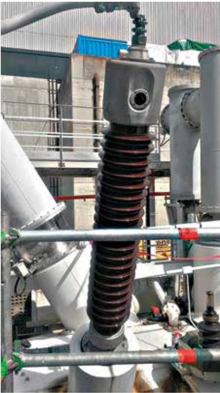
Figure 1. Oil-air bushing
